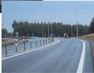
Early research indicates that where the opposing traffic streams are separated by means other than a barrier system there is a 25% reduction in accidents. However a more significant reduction in accident rates is achieved using a barrier system and for this reason a safety barrier system will be included in the pilot 2 plus 1 projects.
