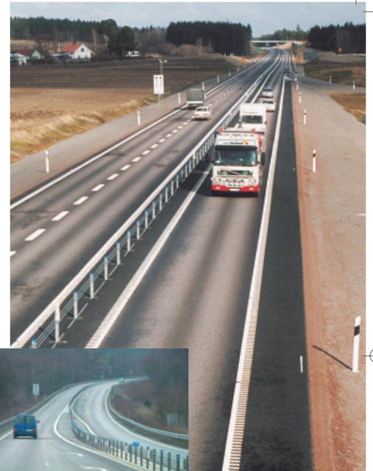
The provision of overtaking sections every 2km reduces driver frustration and the provision of a central safety barrier eliminates imprudent over taking. Provision for right turning movements will only be at designated junctions.
